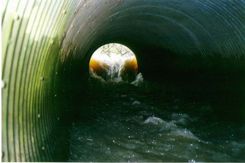
Figure 24. Upstream view through misaligned culvert located in upper Sweetwater HUC. Note the standing wave at the culvert entrance. Surveyed March 2000.
