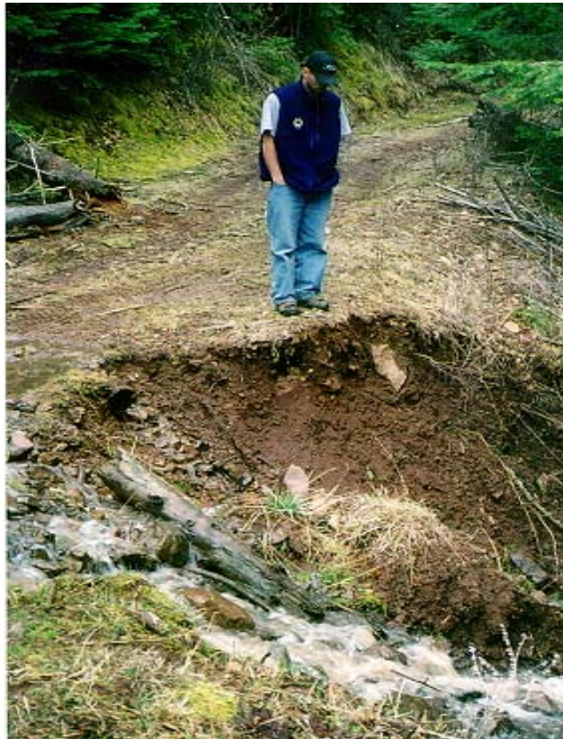
Figure 19. Road slump on native-surfaced road in the upper Sweetwater HUC. Slump attributed to lack of culvert/saturated road fill. Surveyed March 2000.
