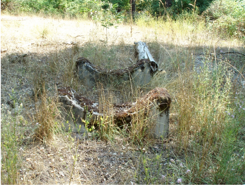
Figure 2; Concrete support saddles for creosote air-lift pressure tank, Richardson Saw Mill site, TU 45.
