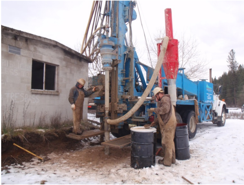
Figure 2. Drilling MW-3 adjacent to Power House
