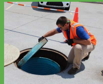
Inspecting a containment sump
