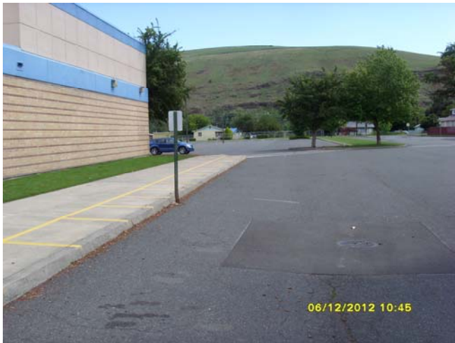
Photo: Stormwater drywell in front of elementary school.
