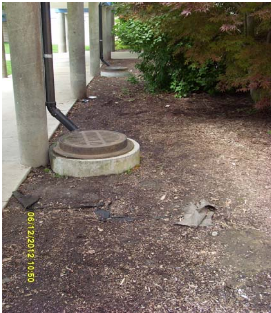
Photo: Roof drains on elementary school building.
