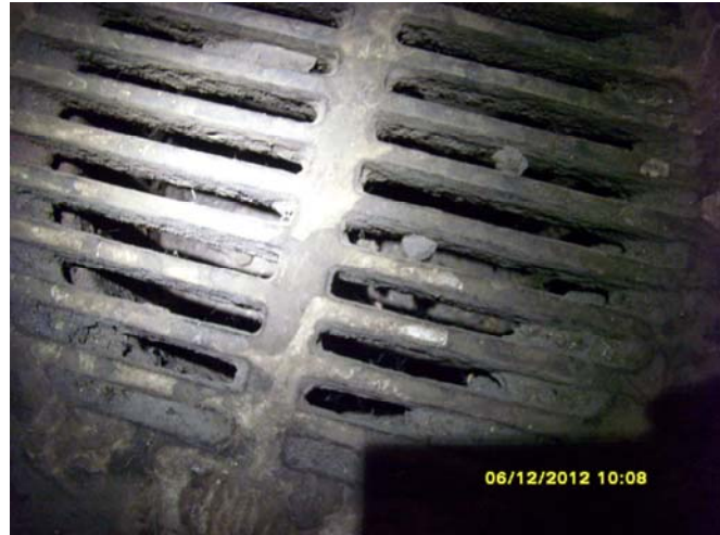
Photo: Looking into equipment bay floor drain.
