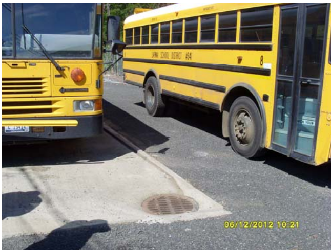
Photo: Bus wash area and drain cover on cement pad.
