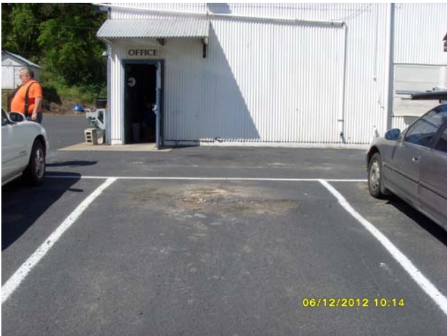
Photo: Looking west at parking space under which the facility representatives think the drywell is located.
