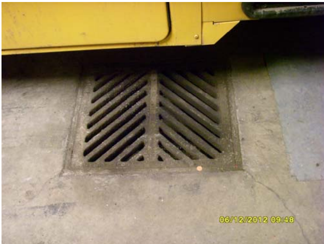
Photo: Floor drain in bus bay.
